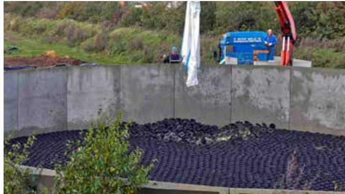
Hexa-Cover® Floating Cover Big Bag delivery and installation:
