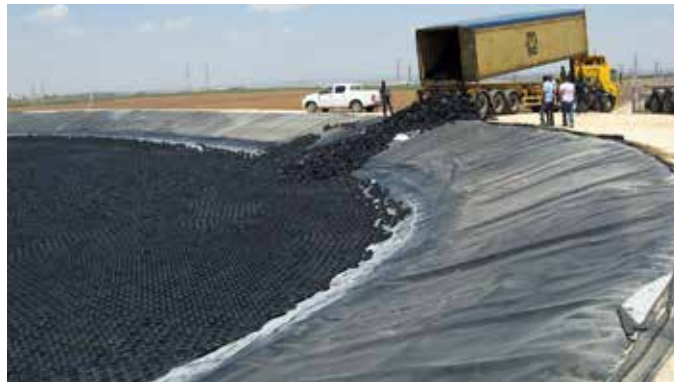
Hexa-Cover® Floating Cover BULK delivery and installation:
