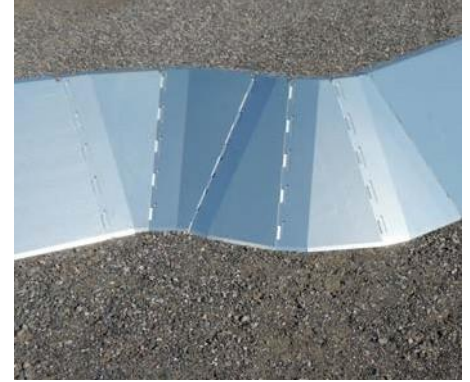
3. When needed use corner sections
