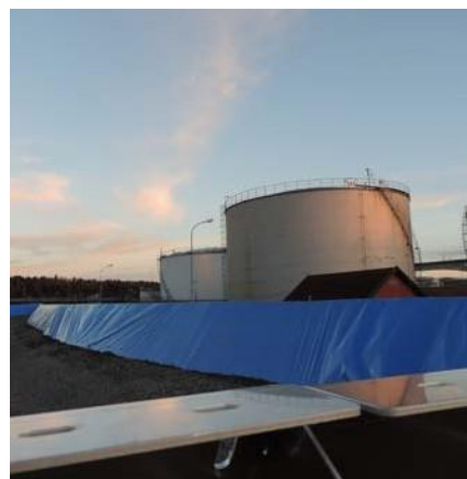
Photo shows the barrier H150 from the water side.
