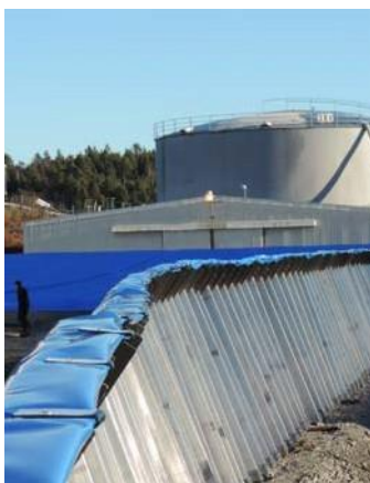
The double folded membrane is fixed with the clips. After clipping fold down the edge and fix the membrane to the ground.
