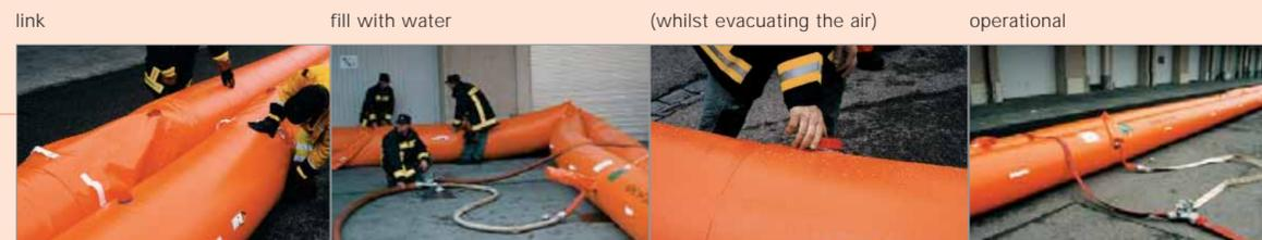
Especially in storms and floods, fast assembly and erection of a dam is crucial. By stacking an additional tube the hold back capacity can be increased quickly and easily in case of an emergency.
